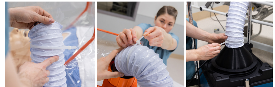
Figure 8: Elbow and duct connection
